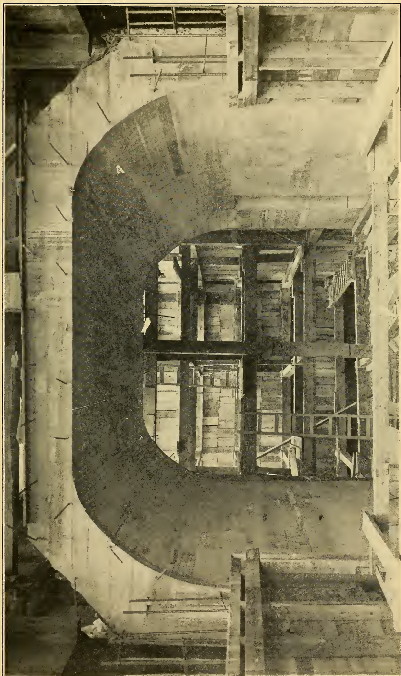
PLATE 7.—TYPICAL SUBWAY SECTION — MAVERICK SQUARE
